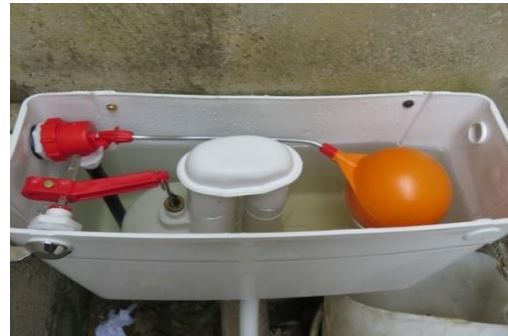
Cistern with syphon flushing device installed
